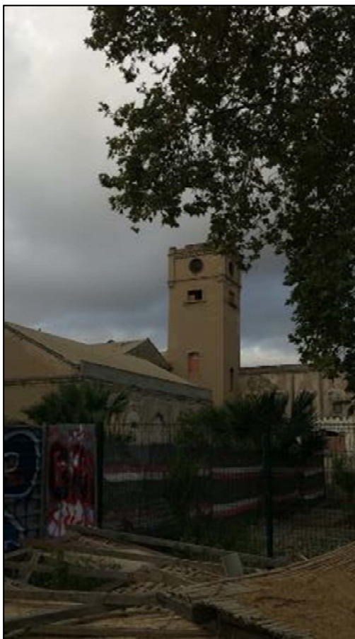
2. Exteriors del complex industrial de Can Ricart.
